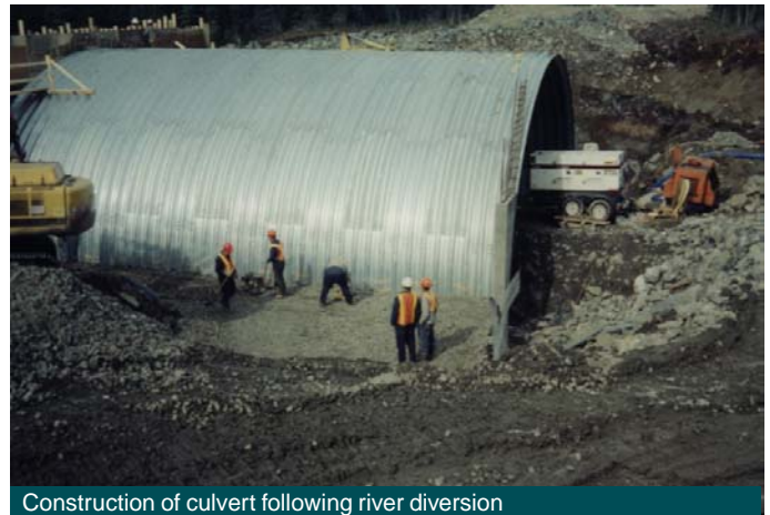
Construction of culvert following river diversion
