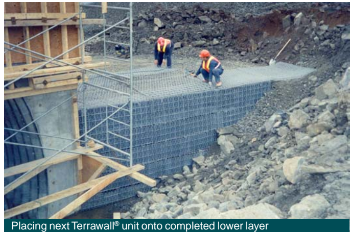
Placing next Terrawall® unit onto completed lower layer
