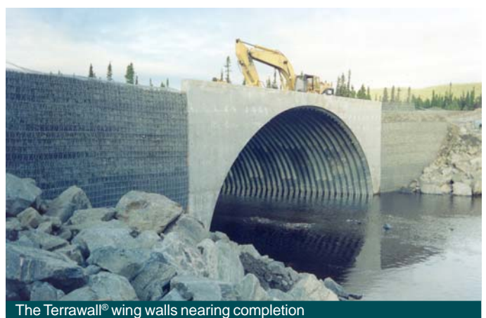
The Terrawall® wing walls nearing completion
