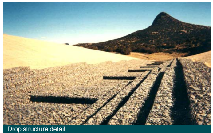
Drop structure detail
