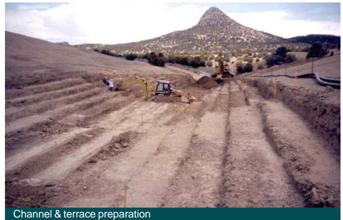
Channel & terrace preparation
