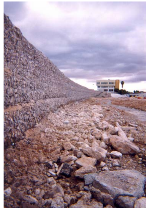
Completed Terramesh® structure
