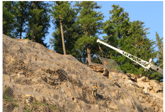
Installation of Maccaferri HEA Panels
