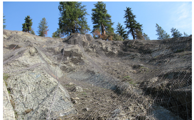
Maccaferri HEA Panels Installed
